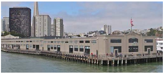
Prologis used PACE to finance lighting upgrades, HVAC, and solar PV at its corporate headquarters in San Francisco. The upgrades saved Prologis 32% in energy costs.
