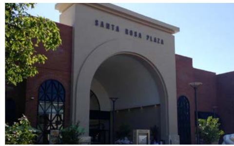
Simon Property Group chose PACE for the Santa Rosa Plaza shopping center, which made use of a $463,000 assessment to finance a cool roof.
